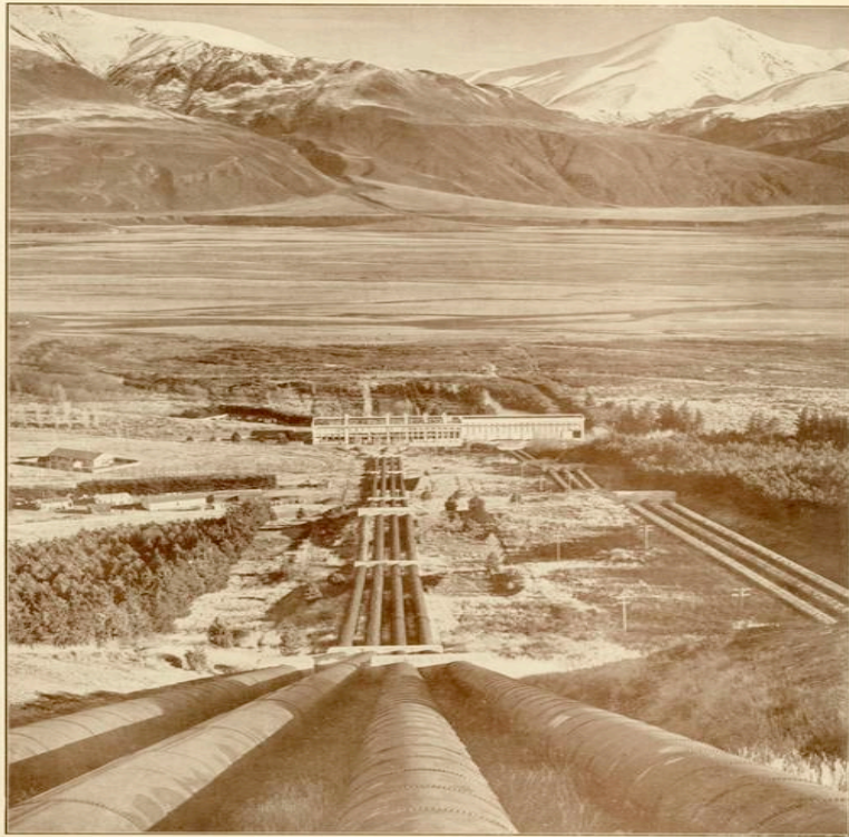
The Lake Coleridge Hydro-Electric Plant, showing the Rakais River, Tail Race, Power House and Pipe Lines. (65 miles west of Christchurch)
